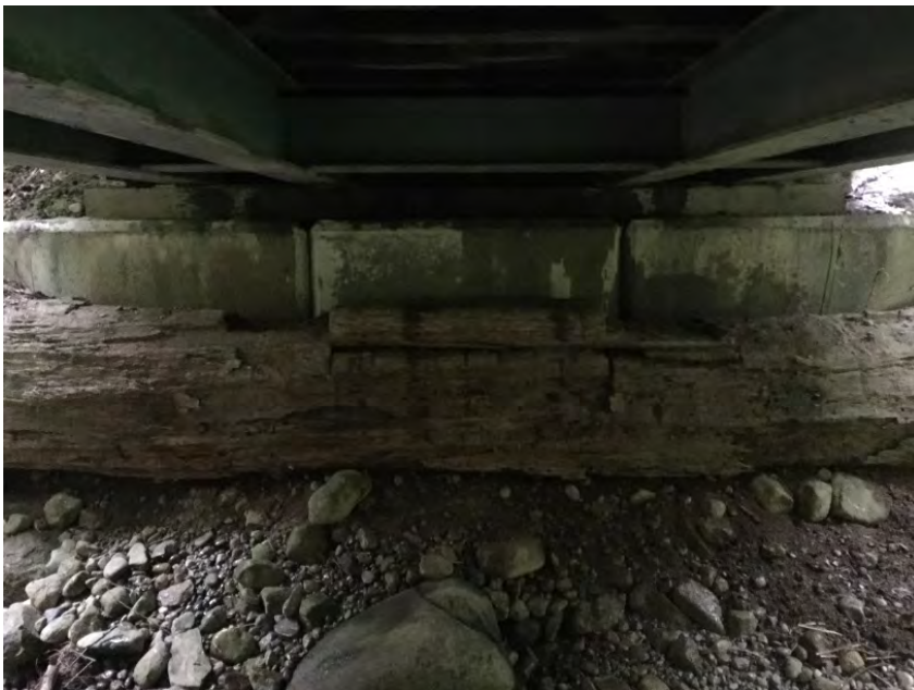
Left Bank Abutment when facing downstream
