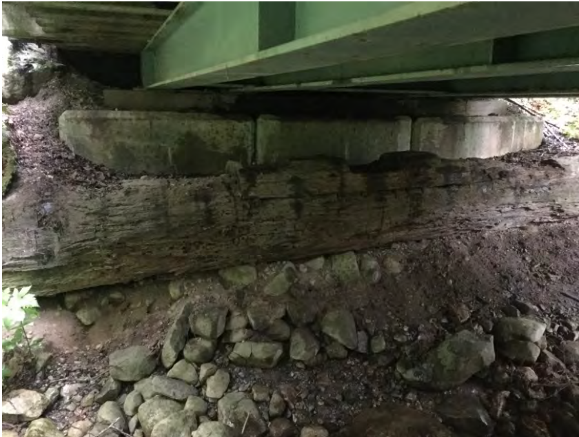
Right Bank Abutment when facing downstream
